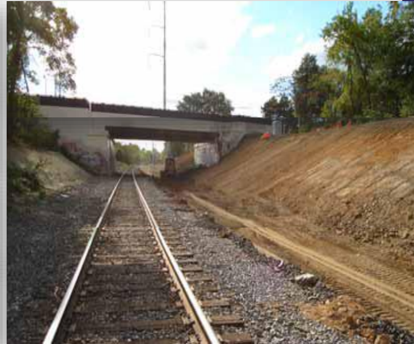
Staged track lowering to maintain rail service
