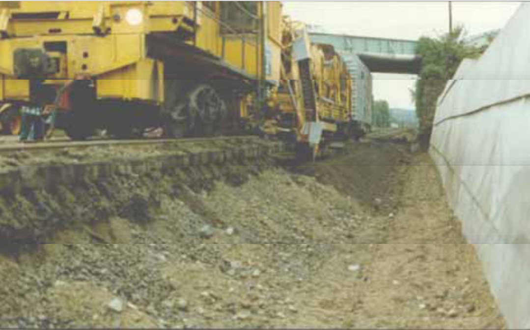
Under-cutting and lowering existing track for additional vertical clearance
